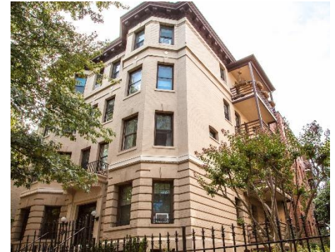
Lambert (17 apartments) - 1791 Lanier Place, NW (Lanier Heights)
